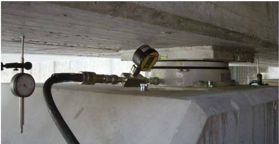
Weighable pot bearing Prébois viaduct – Switzerland
