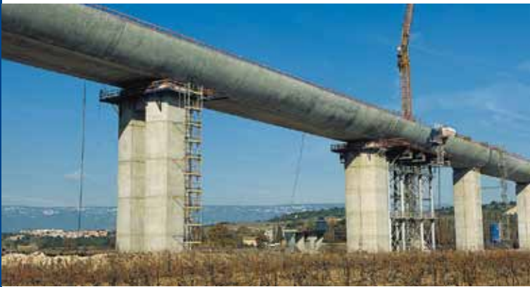
Vernègues viaduct, Mediterranean TGV line – France
