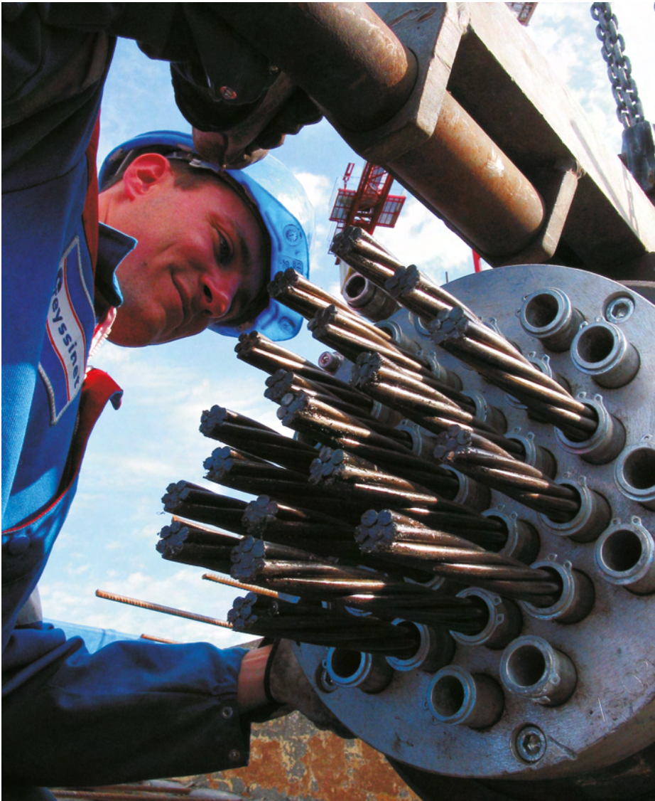
Sioule Viaduct post-tensioning
