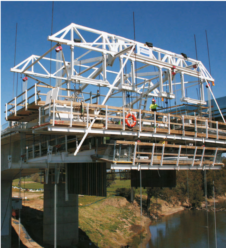
Sheahan Bridge, Australia: above and right, form traveller
