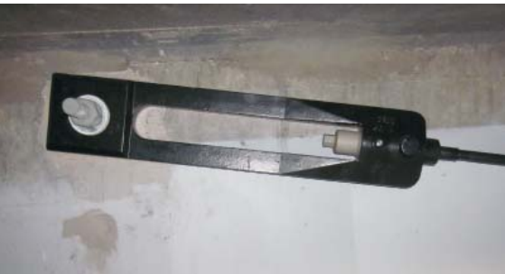
1R15 anchorage in final configuration
