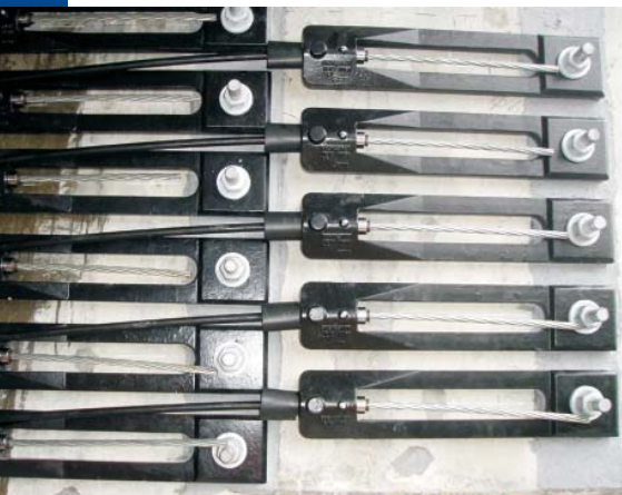
Live ends before stressing
