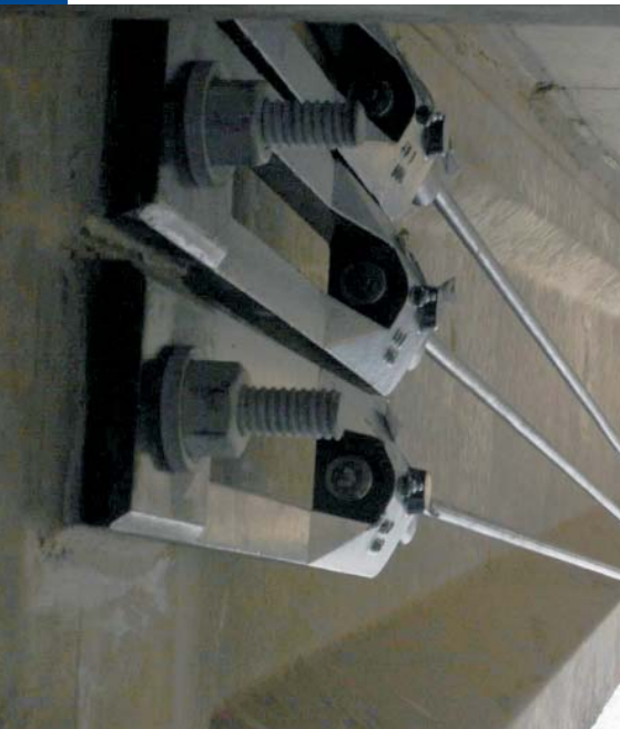
1R15 anchorages stressed
