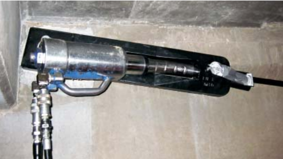
Stressing of the 1R15 anchorage with curved nose and monostrand jack
