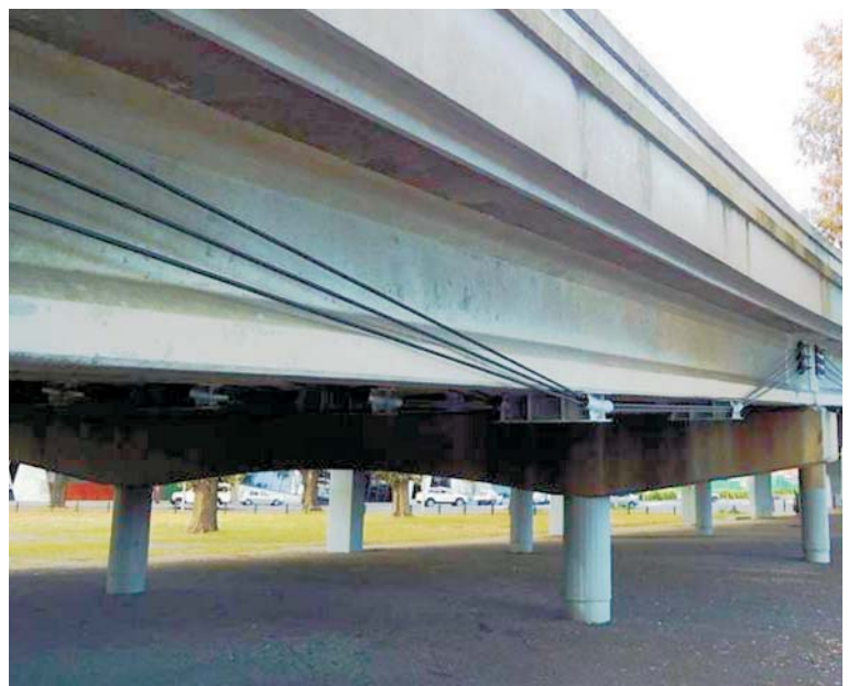
Southern Link Upgrade, Melbourne, more than 2000 No of 1R15 anchorages installed
