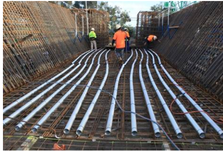
Fig. 7. Prefab installation of Bottom ducting
