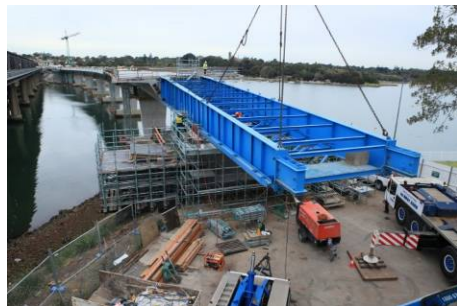
Fig. 16. Launch nose dismantled by section as it passes over Pier 9
