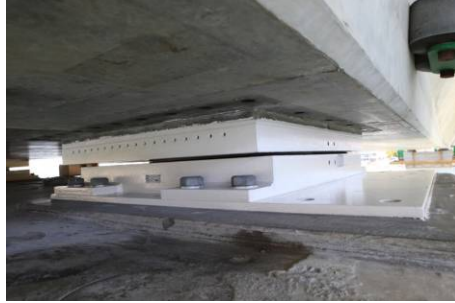
Fig. 23. Bearings completed: shifted, bolted and grouted on their permanent position.
