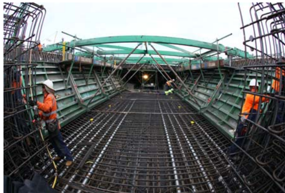
Fig. 6. View of the bottom section of segment being installed
