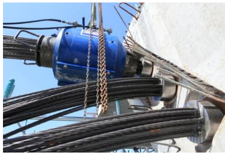
Fig. 11. Stressing continuity tendons from Segment 1
