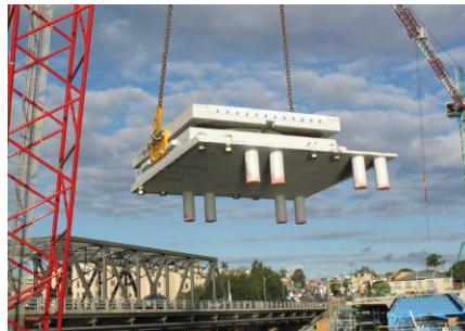
Fig. 20. Bearings being lifted on top of pier
