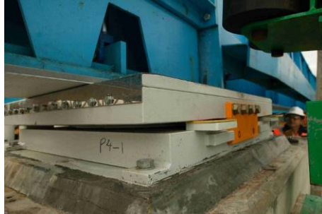
Fig. 21. Bearings in temporary position. The launch nose slides over it.
