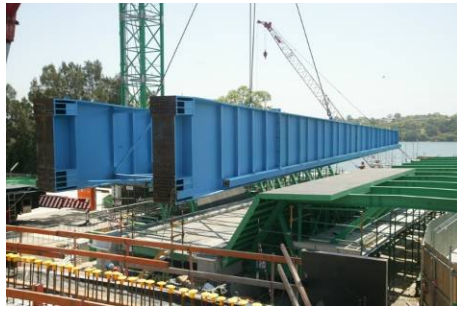
Fig. 15. Launch nose fully assembled and lifted into the casting bed
