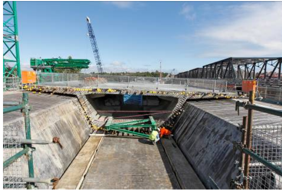
Fig. 4. General view of the inside of the casting bed.
