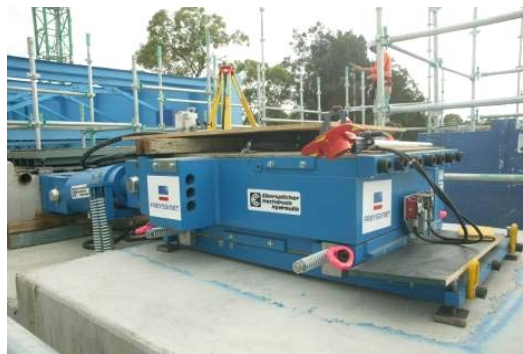
Fig. 18. Eberspächer during installation on TP1
