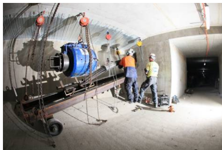
Fig. 12. Stressing continuity tendons from the diaphragm inside the box girder
