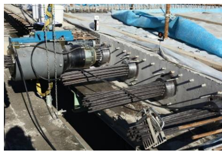
Fig. 9 .Stressing Jack threaded on top tendons
