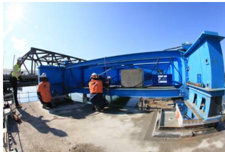
Fig. 14. Launch nose has just been jacked up onto launch pot bearings.
