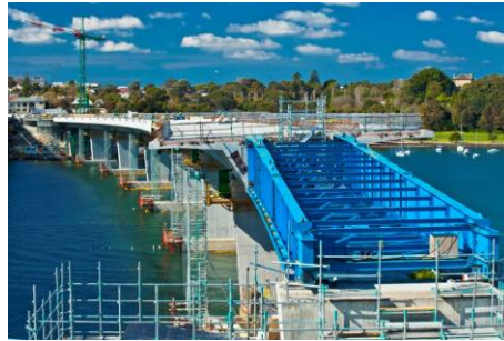
Fig. 13. Launch nose at the last launching pier P9
