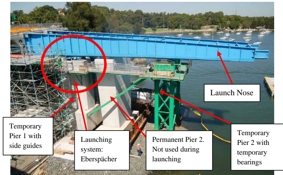
Fig. 19. Launching system setup
